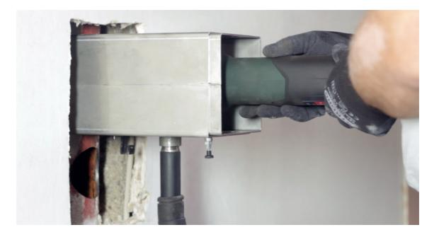
Our PCS System comes equipped with an additional Sleeve Cutting Module, which allows for precision cuts above purtruding tiles and concrete floors. Sewage pipes can now be installed right from the shortened sleeve and laid flush across the floor.
